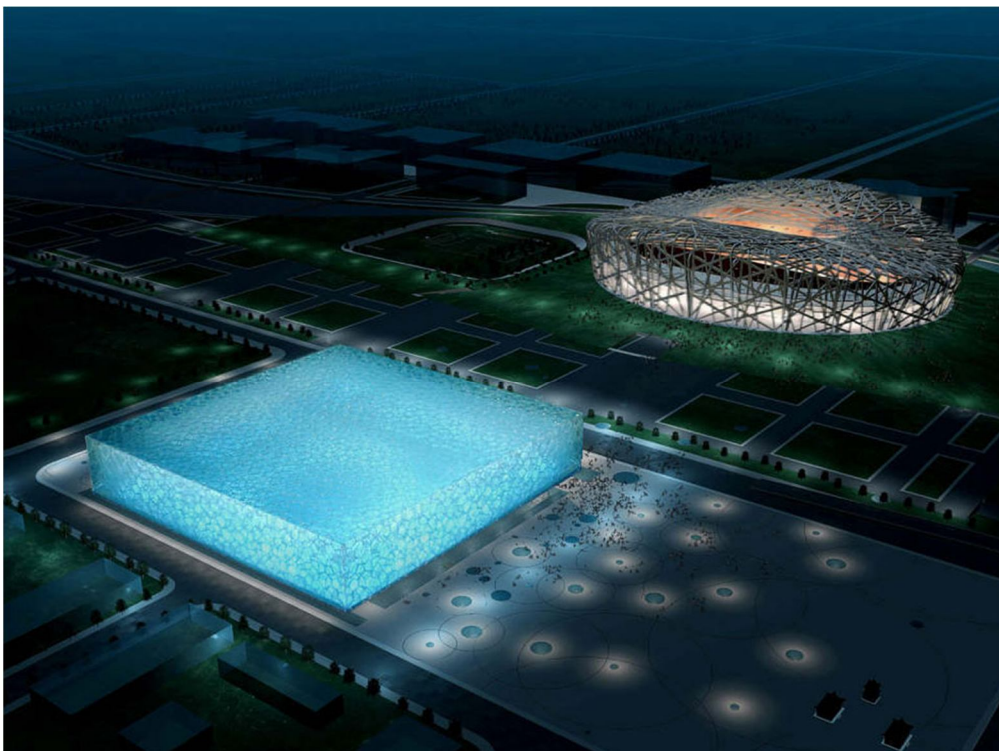
National Stadium (right in the photo) and National Aquatics Centre (left in the photo) at night
